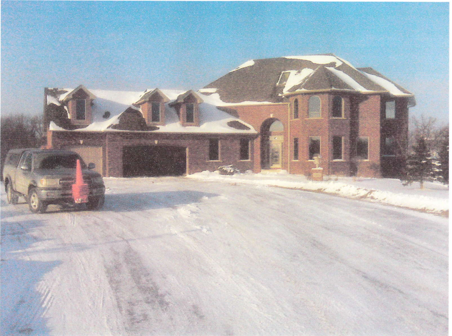
View from South side of house (North Point Drive Cul de Sac side)
